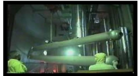
The hairpin heat exchangers of the boiler in MAPS-1 had developed leakage in the tubes. Subsequent to detection of steam generator tube leakage, replacement for all boiler hairpin heat exchangers was carried out successfully in MAPS PHWR units. Based on detailed
