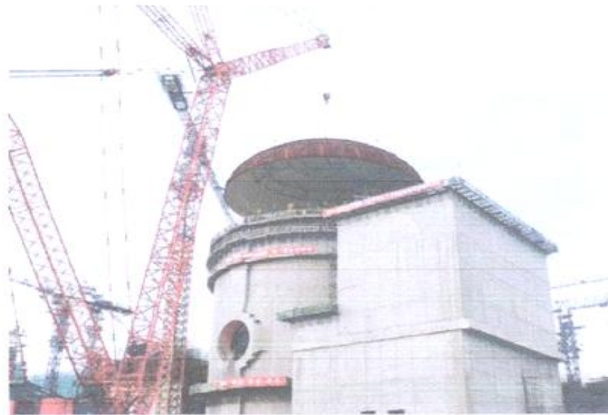
Installing the lid on Ningde 3 (Image: CNECC)
