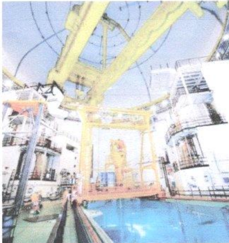
Fuel loading operations at Qinshan II unit 4 (Image: CNNC)
