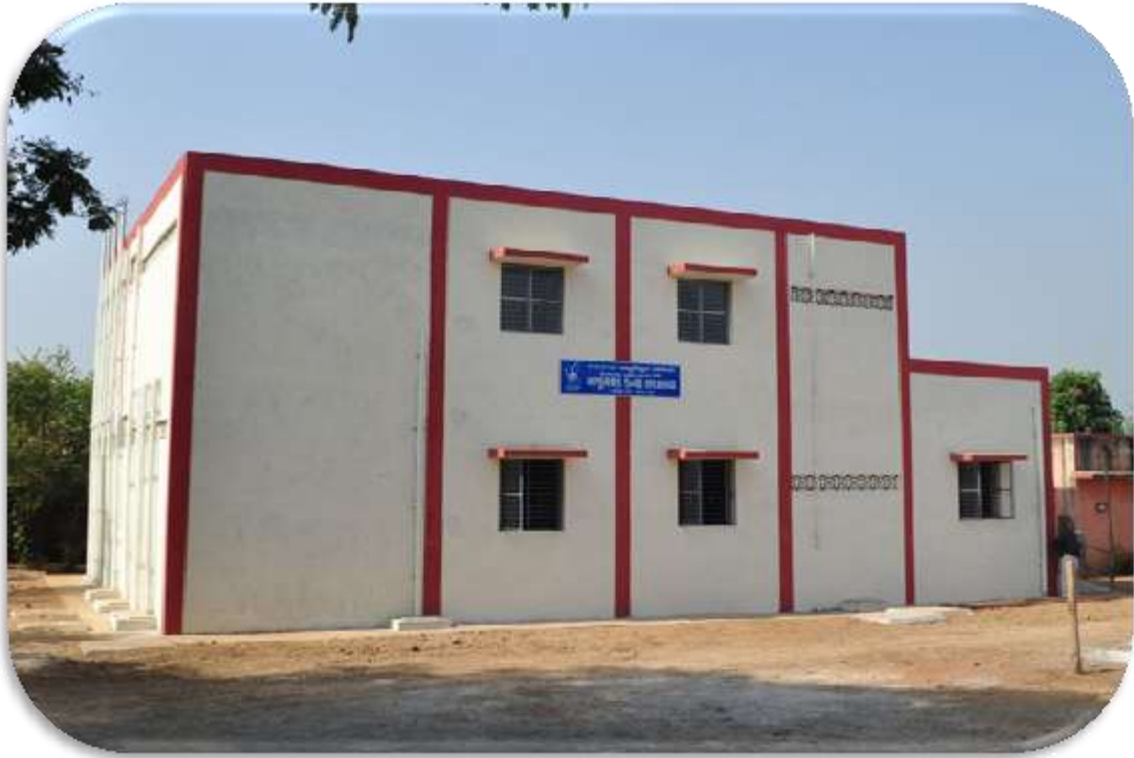
Exterior view of Anumathak Kanya Chhatralaya at Shree L H Bhakta Sarvjanik High School, Ghata
