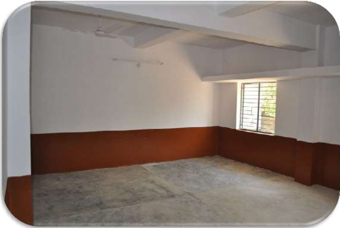
Room facilities in the hostel building.
