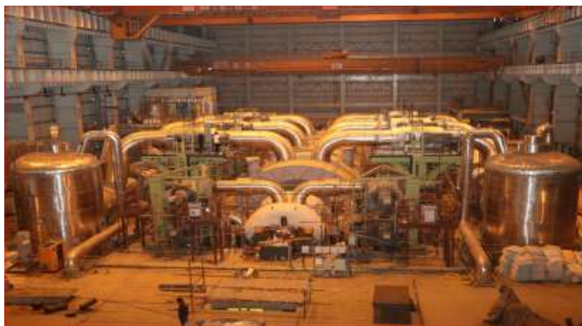
TG on barring gear in KAPP-4
