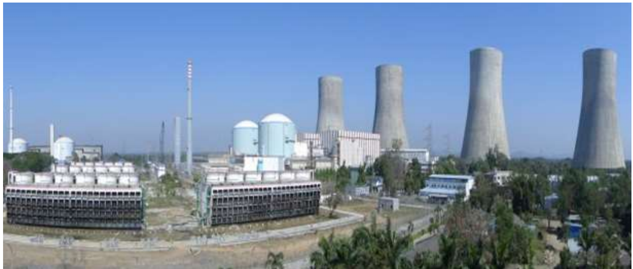
Overall View of Kakrapar Site
